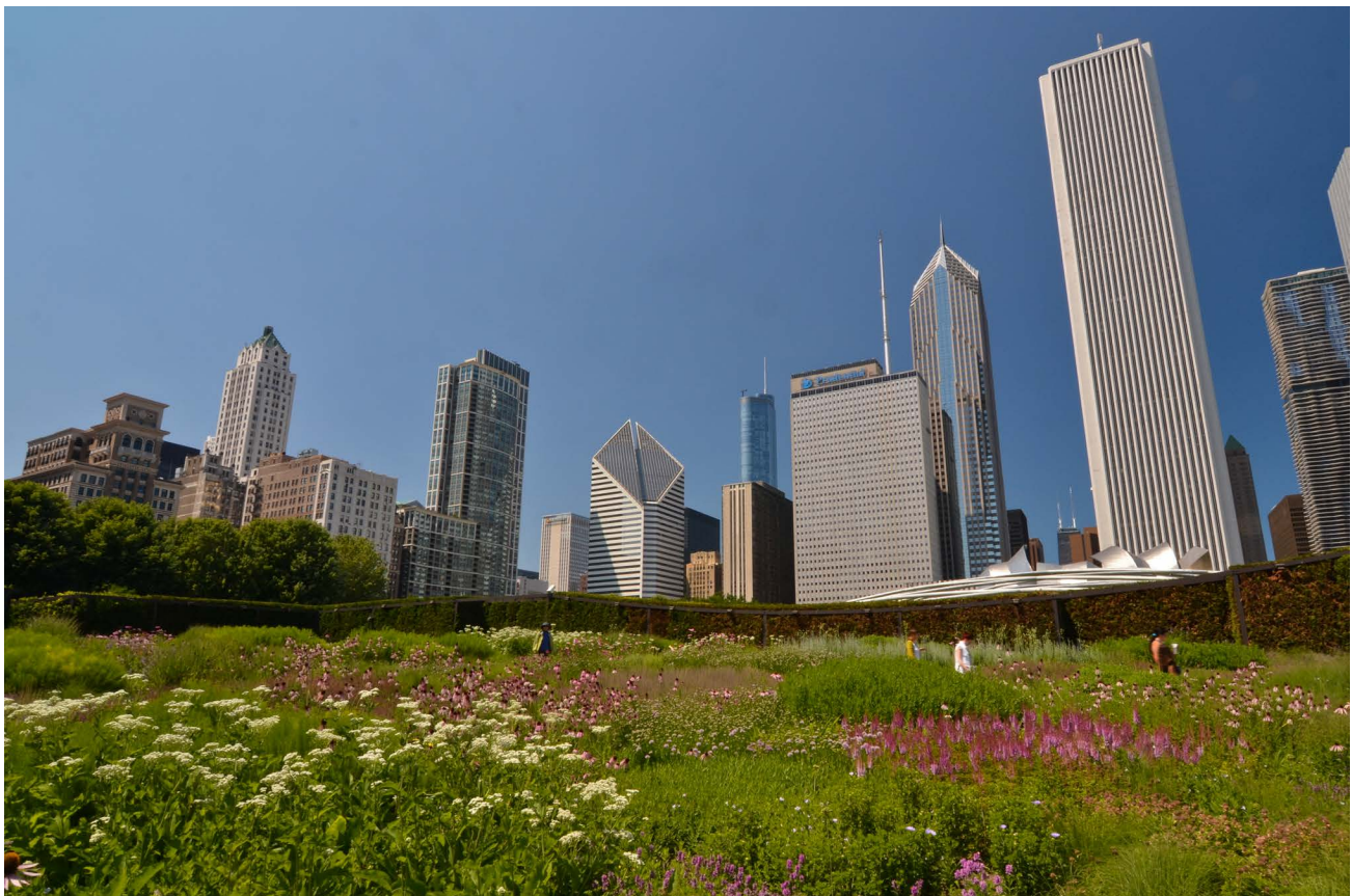
Figure A4 | Green Roof Atop a Parking Garage and Rail Yard in Illinois That Helps Slow Stormwater Runoff
