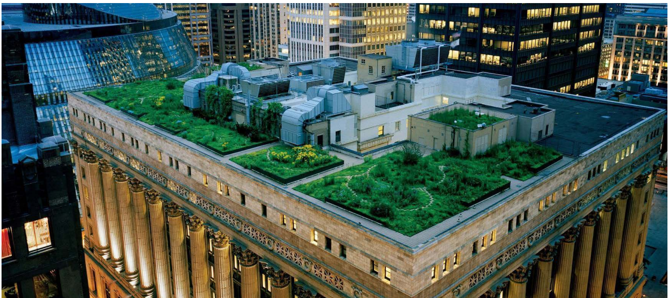
Figure 6.2 | Green Roofs Help Control Urban Flooding While Also Reducing Heating and Cooling Needs for Buildings
